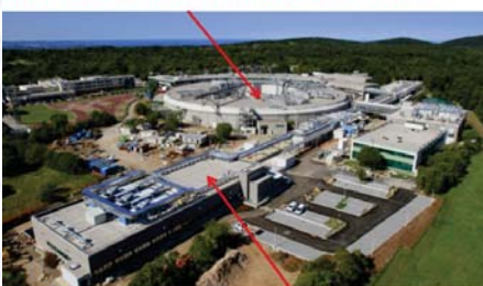
FERMI 1.5 GeV seeded Free Electron Laser Facility
